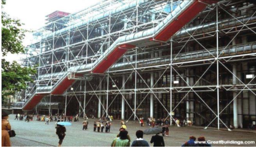
Fig (6) shows the effect of technology on construction in the architectural formation of the buildings of Pompidou cultural center- Paris-France. Designed by the architects (Rogers and Piano)
