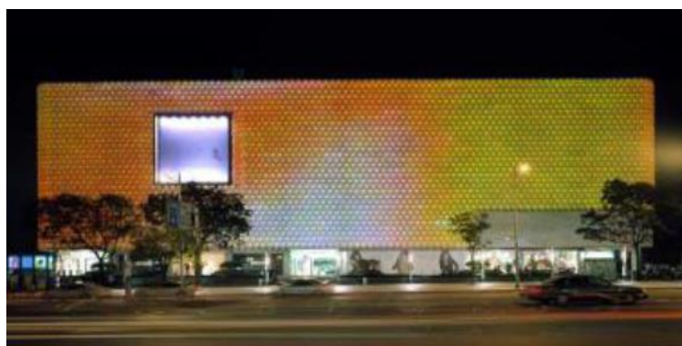
Fig (11) The use of LED. Technic in the outer interfaces of the Korean mall at Seoul city- south Korea- 2003,2004. Designed by UN Studio.
